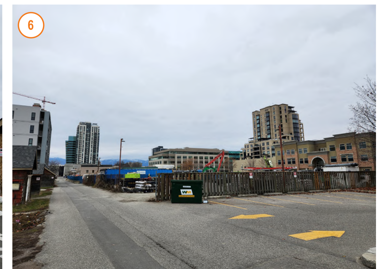
View facing Southwest from the parking lot of the building next door
