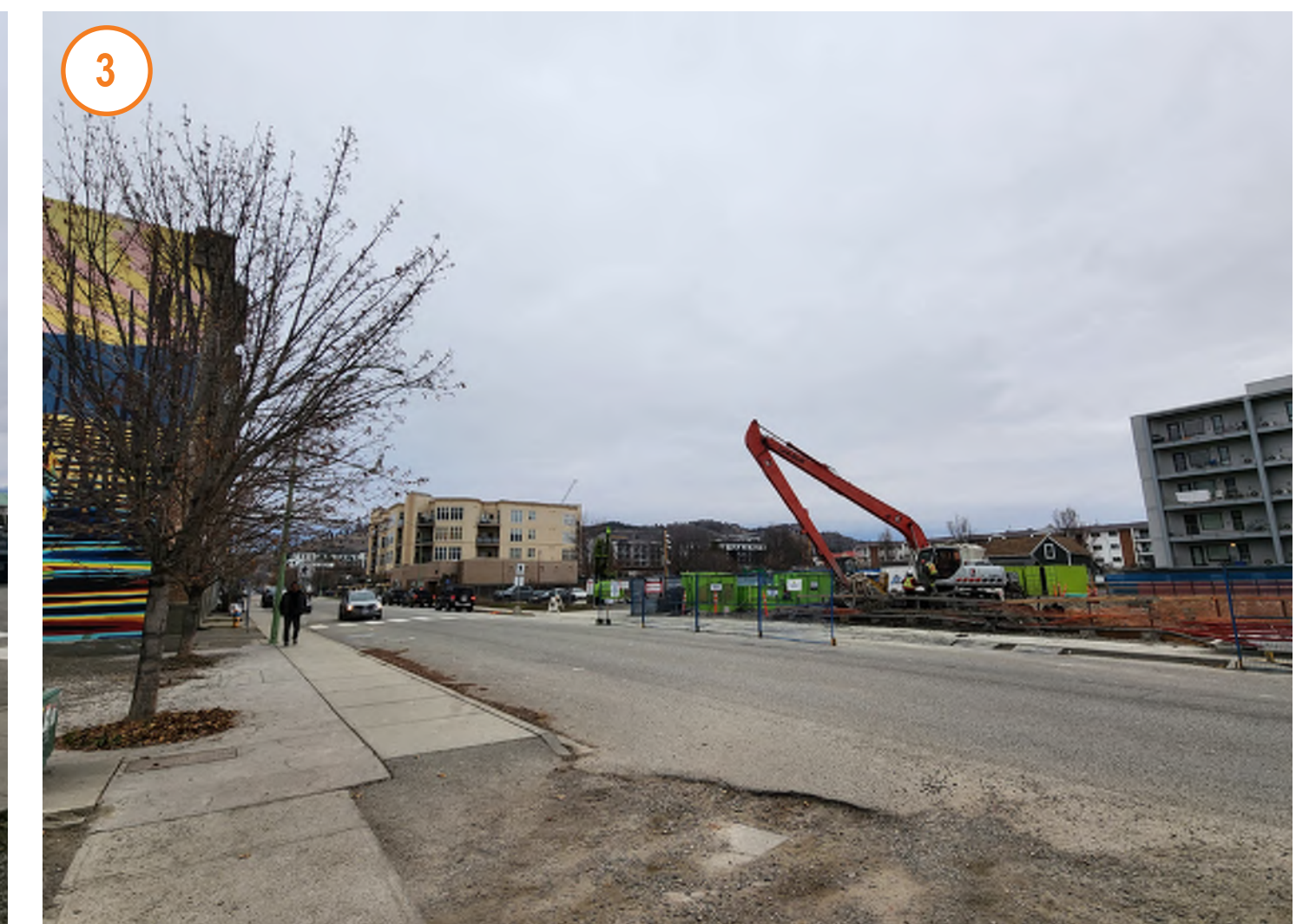
View facing North from the parking lot across UBCO downtown development
